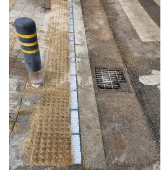
Filling the gaps with silica sand
